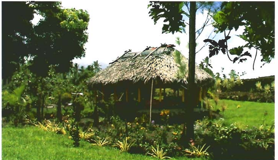
Many Samoans still prefer the natural ventilation of the open-air "Fales" to the introduced wood or brick house.
